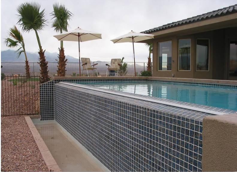
Place top track on tile between 2-3 inches from the top on the 45 degree slope of the outside edge of the vanishing edge.
