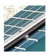
Bond Beam is slanted same as side bond beam. Slant area is 1/2" to 1" higher than side of bond beam.
