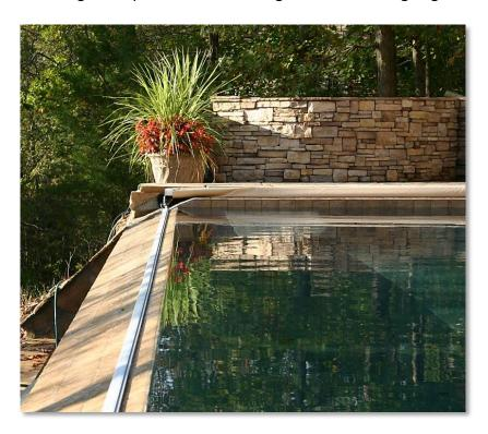
Note spacer under the track. Turn so that corner is pointing away from track. This allows water to flow around and under the track.
