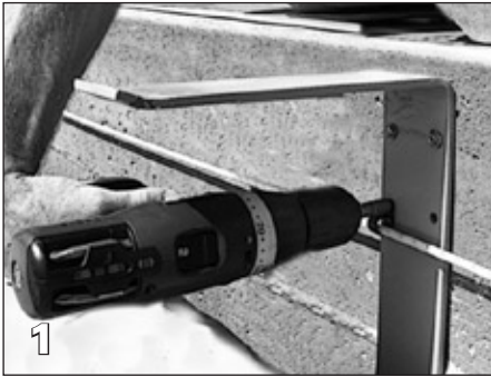
1 Attach the brackets of your choice (ordered separately) to the back wall of the housing 1 in below the top of deck.
