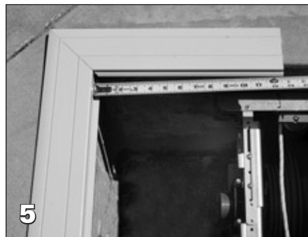
5 Measure and cut the lid panels (X0048), C-cap (X0053), and hinge attachment (X0940) approximately 1/4 in shorter than the actual width to the inside of the lid end supports. This allows the cut cover to attach to the ends of the lid panels to cover any cuts.
