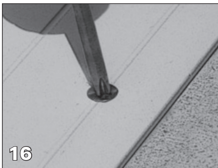
16 Place assembled lid over the housing and screw it into place using the 1 x 1-3/4 stainless steel screws (A2209).
