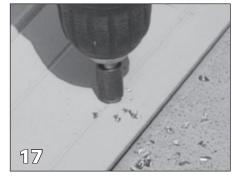
Countersink the drill holes in the hinge.
