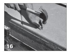
Remove the lid and hammer the plastic anchors (A1706) into the holes.
