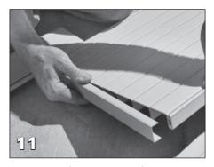
Measure and cut motor and non-motor lid ends to fit. Attach the cut cover pieces (M9363) to both sides of the motor and non-motor end lid.
