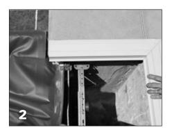
Set the lid end support (A2429) in the ends of the housing in order to get an accurate measurement for the lid panels.
