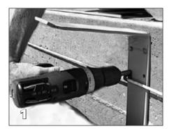
Attach the 97 degree angled brackets (A2430) to the back wall of the housing 1 in below the top of deck.
