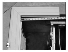
Measure and cut the lid panels (X0048), C-cap (X0053), and hinge attachment (X0940) approximately 1 1/4in shorter than the actual width to the inside of the lid end supports. This allows space for the cut cover and lid wedges to attach to the ends of the lid panels to cover any cuts.
