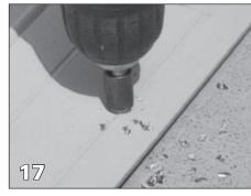
Countersink the drill holes in the hinge.
