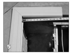
Measure and cut the lid panels (X0048), C-cap (X0053), and hinge attachment (X0940) approximately 1 1/4in shorter than the actual width to the inside of the lid end supports. This allows space for the cut cover and lid wedges to attach to the ends of the lid panels to cover any cuts.
