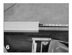
Measure and cut the lid hinge (X0939). Measure from one lid end support to the other.
