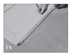
With the lid completely assembled, set it over the housing. Next, mark and drill holes through the lid hinge approximately every 18 inches. Drill the holes into the deck through the holes in the lid hinge
