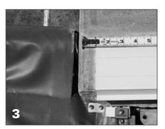
Mark and cut the front side of the lid end supports leaving at least 1 in of flat surface between the coping edge and the lid end support.
