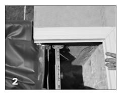
Set the lid end support (A2429) in the ends of the housing in order to get an accurate measurement for the lid panels.
