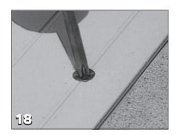
Place assembled lid over the housing and screw it into place using the 1 x 1-3/4 stainless steel screws (A2209).
