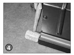
Use a rubber mallet to tap the sections together if necessary.
