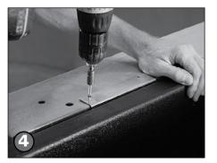
Fasten the "z" channel bracket (3, M9345) to the top of the pool wall using 1" tek screws.
