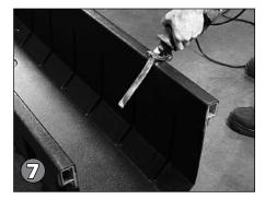
Cut off excess box with metal cutting blade. Housing should be 4 feet longer than the track space. Fit the polymer end piece with junction box (3, A2401) into the motor end of the housing.
