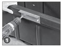
Install the "z" mounting brackets (3, M9345) on the lip of the polymer housing every 24-26 inches. Fasten each section in place with 1" tek screws (1, A1700).
