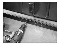
Fasten both splices into place with two 1" tek screws (9, A1701) per splice. Repeat this process to complete the assembly of the polymer housing.
