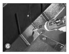
Fasten the sections together from the inside of the housing to the outside with six 1" tek screws. Repeat this process to assemble the full length of the polymer housing.
