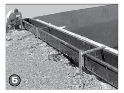
Drive the steel stakes into the ground next to the housing. Level the housing from front to back and fasten the stakes to the housing. The motor and non-motor end are supported with additional stakes, support braces (5, M9788) and feet attachments (7, M9235) see SIDE VIEW - Housing End Support, below, right.
