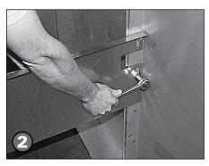
Place polymer housing support brackets (4, M9787) 14-1/4 inches below top of pool wall (See Side View, bottom of page), cutting braces as necessary. Bolt into place using wall joining hardware supplied by the pool wall manufacturer
