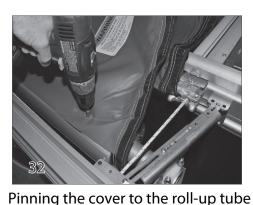
Using a self tapping screw (33), line the cover up straight as it comes out of the track and pin the cover to the roll up-tube on both sides.
