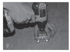
While holding the guide firmly, use a drill with a 3/16" bit to drill through the hole in the guide and through the track. Remove the guide. Do this for the track on both sides of the pool.
