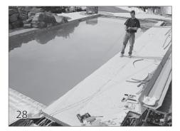
Attaching the Ropes to the Reels The cover must be open when cutting and attaching the ropes. Pull the cover back until the sliders are against the guides. Pull the ropes tight as they come off the pulleys on the mechanism to eliminate the slack in the rope.
