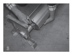
Attach the roll-up tube to the non-motor end of the mechanism using the  $3/8" \times 1-1/4"$  bolts (28) and lock washers (29) provided.
