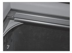
When retainer is being used, the track is normally installed during the cover installation. With the track installed, make sure it is flush with the end wall at the shallow end.
