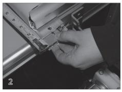
Cut the length of the track on each side of the pool so it will extend 1 inch past the end of the retainer and into the cover box.
