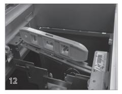
With the brackets on the non-motor end in position, place a small level across the brackets to make sure they are level. Tighten the nylock nuts on the adjustable brackets.
