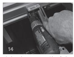
Anchor the non-motor side of the mechanism into the cover box in as many places as possible. Use the appropriate screws and anchors depending on the type of cover box being used.
