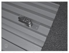
Repeat the same installation steps to install the second lock on the other end of the lid panels. Make sure the locks point toward the center of the lid when in the locked position.
