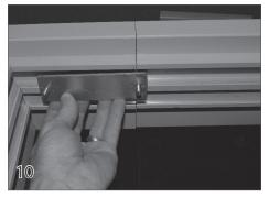
Insert a second QuickAttach anchor plate in the top channel of the riser on the back side of the cover box. Repeat inserting anchor plates on the opposite side of the cover box.
