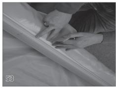
Distribute the slack of the cover evenly between each screw across the length of the tube. Secure the cover to the roll-up tube using #10 x 1/2" SS tek screws (23) every 2-3 feet.
