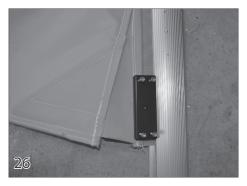
Use a drill with a 5/32" hex bit to tighten the 4 hex-head screws in the stop.
