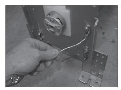
Make the same connection with the #8 copper bond wire that is near the mechanism on the non-motor end of the mechanism.
