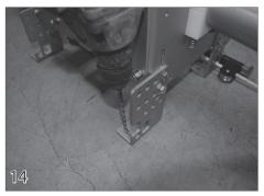
Anchoring The Mechanism Use a 1/4" bit and hammer drill to drill through the mounting holes in the mechanism into the deck.
