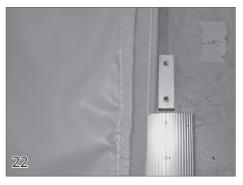
Slide the Stop Plate Support Splice (35) into the track. Line up the holes in the support splice with the holes in the track.
