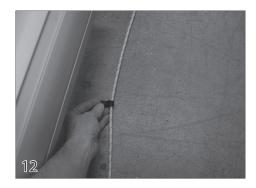
Run the rope from the non-motor end along the pool deck behind the mechanism. The rope should run through the rope loops (15) to keep it from getting caught in the cover. Space the rope loops evenly behind the mechanism.
