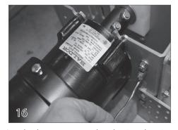
Attach the #8 copper bond wire that is stubbed near the mechanism to the bonding lug on the motor end of the mechanism.
