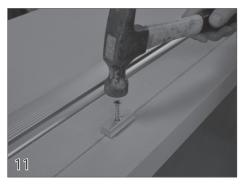
Use a hammer to tap the screw head down until the anchor is flush with the top of the pool deck.
