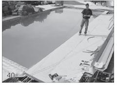
Attaching the Ropes to the Reels The cover must be open when cutting and attaching the ropes. Pull the cover back until the cover is in the fully open position. Pull the ropes tight as they come off the pulleys on the mechanism to eliminate the slack in the rope.
