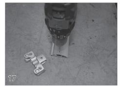
Use a drill with a 5/32" bit to drill through the track where it was marked in step 16.
