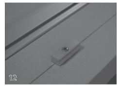
Using a #3 Phillips bit, tighten the screw to secure the snap-lock to the pool deck.
