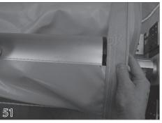
Attaching the Cover & Bonding Wire Make sure the webbing continues straight as it travels from the track to the roll-up tube. Attach the cover to the roll-up tube using #10 x 1/2" SS tek screws (23). The first screw on each end of the tube needs to be 3 inches from the end of the tube. As the cover rolls up on the tube, the webbing will be rolling up over the end casting.
