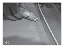
Using a utility knife, carefully cut a slit in the webbing long enough for the magnet to be slid through. Be careful not to cut through the bottom layer of webbing.
