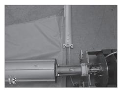
On one side of the cover, pull the rope as it comes out of the track as you feed the cover into the track. Keep pulling until the webbing is in the track a few inches. Having the webbing on one side of the cover in the track will help with the installation of the leading edge bar.
