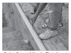
Fasten Encapsulation in Place Place the encapsulation back over the holes and anchors. Secure the encapsulation to the pool walls by inserting a hex head screw and tightening with a drill. Tip: Install track and spacer in the encapsulation to help the encapsulation and corners line up straight while it is being secured to the pool wall.
