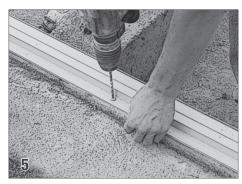
**Drill Holes in the Wall** Drill through the back flange of the encapsulation 2 1/2" deep. These holes should be placed every 24 - 30 inches.
