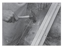
**Tap in Anchors** Move the encapsulation back a few inches to expose holes. Insert plastic anchors into each hole.
