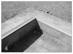
Miter the Corners Begin at the end of the pool opposite the cover mechanism. Miter cut a 45 degree angle on the ends of two lengths of encapsulation. Place them together on the corner to form a 90 degree corner. Make the same cuts for the other corner of the pool. Continue placing lengths of encapsulation around the rest of the pool. Cut the encapsulation so it will extend 1 inch into the cover housing.
