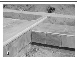
Place the Encapsulation If encapsulation is installed before the tile, overhang the encapsulation 1/2" into the pool aligned with the string line. If the tile has already been installed, place the encapsulation flush with the tile.
