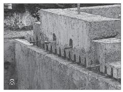
Optional Raised Wall with Pocket Holes Pools with a raised wall need a cavity large enough to accept the encapsulation (3"x 2") and should have pocket holes formed to allow it to the encapsulation to be screwed into place.
