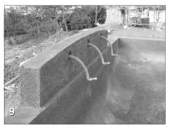
**Optional Raised Wall** Pools with raised walls can also be formed with a three inch ledge. The encapsulation is anchored to the ledge, allowing stone to be set in place on top of the encapsulation. It is important that the track and spacer be inserted into the encapsulation to prevent it from collapsing.
