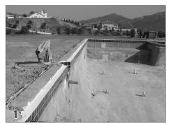
Mortar A Level Mounting Bed Mortar the top of the gunite walls so they have a 3" min flat, straight and level surface for the encapsulation to be mounted to.
