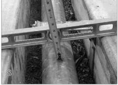
With the mechanism and tube assembled and set in place in the housing, check the roll-up tube for level. This is crucial to proper operation of the cover. Position a level across the housing. Measure from the roll-up tube to the bottom of the level on both the motor end and non-motor end of the mechanism. Adjust height of the non-motor end feet if needed to level the roll-up tube.
