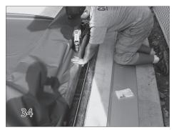
Attaching the Cover & Bonding Wire
