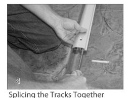
Before splicing the sections of track together, file all track ends thoroughly,
