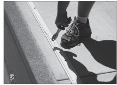
Hold the wire with some pliers and pull the rope down the length of the track toward the end of the pool.
