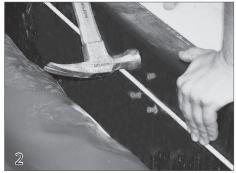
Remove the bracket and insert plastic anchors in each of the holes. Tap the anchors with a hammer so they are in the hole completely.
