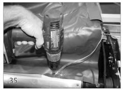
Lay the bond wire on top of the cover fabric. Secure it to the roll up tube using a tek screw (42). Distribute the slack of the cover evenly between each screw across the length of the tube. Secure the cover to the roll-up tube using tek screws (42) every 2-3 ft. When attaching the cover to the tube, do not use folds or pleats.
