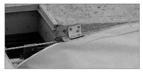
(6) OPTION: Recessed horizontal track sloped into the box. Purchase set of curved tracks for housing end of track. Bend begins 15" in front of housing. Make sure top of track is minimum of 1" lower than bottom of lid.
