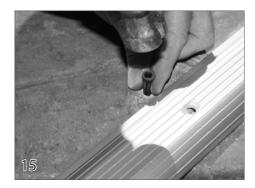
Move the tracks to the side to expose the holes in the deck. Clean the dust from each hole and tap plastic anchors (41) into each one.
