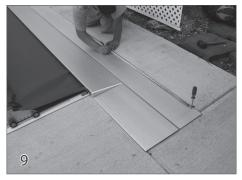
Measure across the hinge to evenly space the screws. Continue drilling and anchoring the hinge in this manner until the entire lid is attached to the deck. If any part of the lid is sticking up, it must be screwed down to the deck. The safety pool cover installation is now complete. Now instruct the home owner using the home owners guide and the checklist on the next page.
