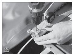
Place a guide feed (23) over the end of the track. Use a 3/16" drill bit to drill through the guide feed. Feed the wheel assembly and cover into the track.
