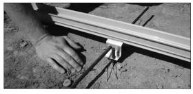
(4.a.) Track staked in place using the optional mounting feet, ready for pour
