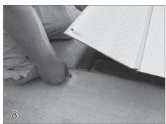
Insert plastic anchors (38) into the holes and tap with a hammer so they are flush with the deck. Fasten the lid to the deck with #12 pan head screws (32). File any sharp edges.
