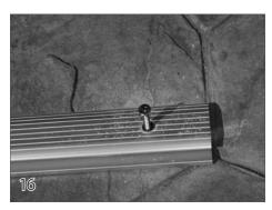
Place the track back over the holes in the deck. Fasten the track screws (34) <u>halfway</u> through the tracks into the plastic anchors. The screws will be fastened completely later in the installation.
