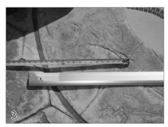
Extend the tracks 18" past the waterline at the shallow end of the pool. Center the pool shape between the pool track where possible. Measure and mark the track length on the deck. Use a chalk line to mark the track location.
