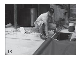
Attaching the Cover Leading Edge Lay the front of the cover in front of the housing. Slide the leading edge through the loop on the front of the cover.
