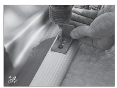
Install a track stop (49) on the end of the track on each track to keep the cover from retracting too far. Run the key switch in the uncover position to roll the cover up on the roll-up tube. Check the cover to be sure it rolls up evenly. The cover fabric installation is now complete.
