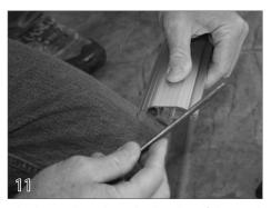
File the track ends on both sides of the pool making sure to round all edges and remove all burrs. This step is extremely important. The cover can be damaged very easily by metal burrs and this damage is not covered by the warranty.
