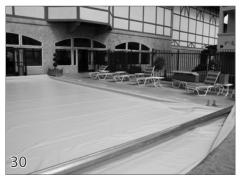
Running the Cover Over the Pool Run the cover over the pool being careful to prevent it from binding in the guide feeds by lifting the cover and helping it into each track the first time.
