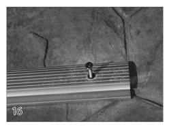
Place the track back over the holes in the deck. Fasten the track screws (34) <u>halfway</u> through the tracks into the plastic anchors. The screws will be fastened completely later in the installation.
