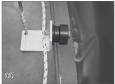
To help the cover roll up evenly, install a cover roller (37) 2-3 inches behind the guide feed. Secure the cover roller to the deck using the screws (15) and anchors (25) provided.
