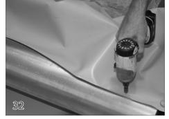
The first two screws need to be 3" from the end of the tube. Distribute the slack of the cover evenly across the length of the tube. Secure the cover to the roll-up tube using tek screws every 2-3 ft. When attaching the cover to the tube, do not use folds or pleats. Operate the cover 6-10 times to make sure it is opening and closing squarely.
