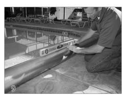
With the mechanism and tube assembled, check the roll-up tube for level. If the deck isn't level, the distance from the deck to the tube should be the same on both ends of the tube.
