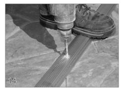
Attaching the Tracks to the Deck Place the tracks into position on the deck in the marked positions. Make sure that the tracks run completely straight on both sides of the pool. Drill through the pre-drilled track holes into the deck. Drill at least 3" deep.
