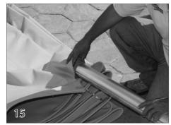
Attaching The Cover Leading Edge Lay the front of the cover in front of the mechanism. Slide the leading edge through the loop on the front of the cover.
