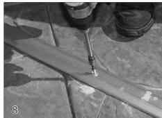
Complete the fastening of all track screws flush on the top of the track. Clean concrete dust from track and pulley end cap. Make sure ALL screws are flush with the top of the tracks.
