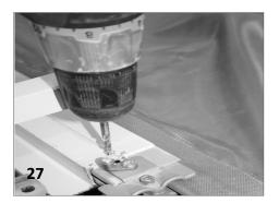
Install a bonding lug on top of the guide feed. Drill through the center of the encapsulation and track. Insert a 10-32 x 1-3/4 screw (40) and nylock nut (27). This step is very important. This will prevent the track from sliding into the cover box during the operation of the cover system.
