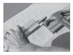
Tap the splice pins (37) into one end of the track and slide the center splice (22) into the center channel.
