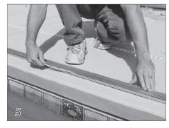
Pull the rope along the water side of the track towards the pulley end cap.
