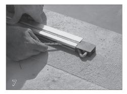
Press the rope into the back side of the track and pull through towards the cover box. Insert the pulley end cap into the track. Repeat this on the other side of the cover.
