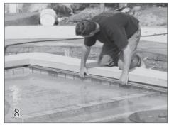
Install the track into the encapsulation with the slider channel facing inside toward the pool.
