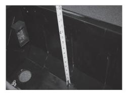
To attach the feet, first measure the distance from the bottom of the cover box to the bottom of the track. (This will determine the height of the mechanism.)
