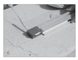
Feed the rope around the pulley end cap. (14)
