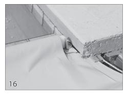
Feed one side of the cover and slider into the track. This will make it easier to insert in the leading edge tube.
