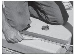
Take a short length of rope outside the track and press it into the rope channel that is closest to the pool. This will allow some rope to remain outside the track for easier pulling of the rope down the length of the track.
