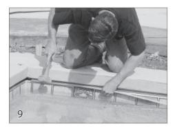
Install the spacer underneath the track to lock the track into the encapsulation.
