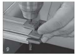
While holding the guide feed firmly, use a 6 inch 3/16" bit to drill through the hole in the guide feed and through the track. Remove the guide feed. Do this for the track on both sides of the pool.
