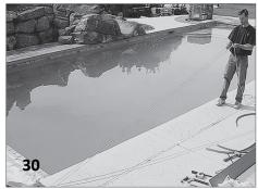
Leaving an extra 6-8 feet of extra rope length, pull on the ropes until the leading edge begins to move forward equally on both sides. Use a lighter to burn the rope where it will be cut prior to cutting it. After the rope has been cut, burn the ends of each rope to keep them from fraying.
