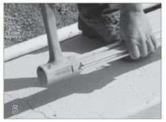
Lay the sections of track on the deck and tap them together using a rubber mallet so the center splice and splice pins interlock with each section of track. It's important that, the splice is tight together so there is not a gap from one track to the next. Slide pulley end cap (14) into the end of the track at that is at the opposite end of the pool from the mechanism.
