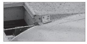
(6) OPTION: Recessed horizontal track sloped into the box. Purchase set of curved tracks for housing end of track. Bend begins 15" in front of housing. Make sure top of track is minimum of 1" lower than bottom of lid.
