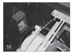
Attach the #8 copper bond wire that is stubbed into the cover box to the bonding lug on the motor end of the mechanism.
