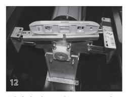
With the brackets on the non-motor end in position, place a small level across the brackets to make sure they are level with the bottom of the track. Tighten the nylock nuts on the adjustable brackets.
