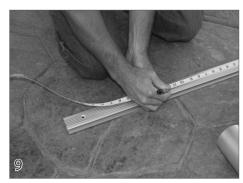
Cutting the Tracks to Length With tracks extended 1 inch into the cover box at the mechanism end, cut the tracks so they extend 18" past the waterline at the opposite end of the pool.
