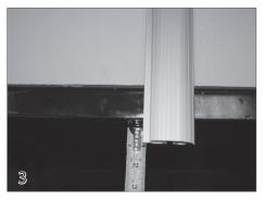
Cut the length of the track on each side of the pool so it will extend 1 inch past the inside edge of the cover box at the mechanism end.
