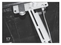
Make the same connection with the #8 copper bond wire that is in the cover box on the non-motor end of the mechanism.
