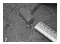
At one end, use a rubber mallet to tap the track sections together.
