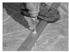
Complete the fastening of all track screws flush to the top of the track and fasten the pulley screw on both sides of the pool. Clean concrete dust from tracks and pulley endcap. Make sure ALL screws are flush with tracks.
