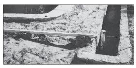
(4.b.) Housing in place mounted on gunite piles ready for deck pour.
