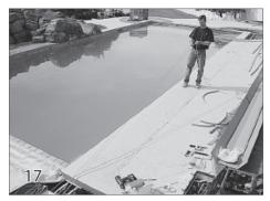
The cover must be open when cutting and attaching the ropes. Pull the cover back until the sliders are against the guides. Pull the ropes tight as they come off the pulleys on the mechanism to eliminate the slack in the rope.
