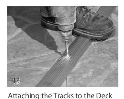
Place the tracks into position on the deck in the marked positions. Make sure that the tracks run completely straight on both sides of the pool. Drill through the pre-drilled track holes into the deck. Drill at least 3" deep. For wood or acrylic decks, pre-drill a 3/16" hole, then use screws to secure the track to the
