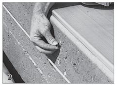
Remove the bracket and insert plastic anchors in each of the holes. Tap the anchors (33) with a hammer so they are in the hole completely.
