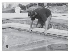
**Install Track in the Encapsulation** Starting at one end, lift the track so it will interlock with the encapsulation. Make sure the track extends 1" into the housing.
