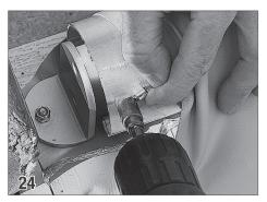
Connect the bonding wire that is attached to the front corner of the cover to the leading edge bar using a tek screw (32). Be sure the screw doesn't interfere with the leading edge insert.
