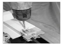
Drill through the center of the encapsulation and track. Insert a  $10-32 \times 1-3/4$  screw (42) and nylock nut (29). This step is very important. This will prevent the track from sliding into the cover housing during the operation of the cover system. (If the encapsulation was cut flush to the inside of the housing, secure the track using a track retainer bracket (23)).
