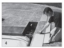
Assembling the Aluminum Lid The aluminum lid will come with each section cut to length. Assemble the lid by sliding the hinge onto the main section of lid.
