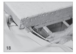
Pull the rope where it comes out of the track as you feed the slider and cover into the track a short distance. The guide feed should not be installed on the cover track at this point.
