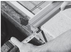
Cut the track so it will extend from the front edge of the coping at the far end of the pool to 1" past the inside of the housing if no encapsulation is being used. When encapsulation is used, it will extend one inch past the inside of the housing, with the track extending one inch past the end of the encapsulation.
