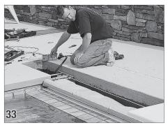
Run the key switch in the uncover position to roll the cover up on the roll-up tube. Check the cover to be sure it rolls up evenly. Run the cover 6-10 times to make sure it opens and closes evenly. The cover fabric installation is now complete.
