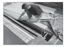
Pull the rope along the back of the housing to the motor side.
