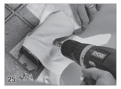
Position the fabric on the leading edge so it is in line with the leading edge support bracket. Secure with a tek screw (32) on the back side of the leading edge. Be sure the screw does not interfere with the leading edge insert.
