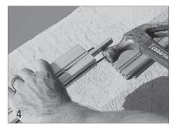
Tap the splice pins (39) into one end of the track and slide the center splice (24) into the center channel.
