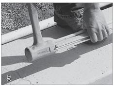
Lay the sections of track on the deck and tap them together using a rubber mallet so the center splice and splice pins interlock with each section of track. It's important that, the splice is tight together so there is not a gap from one track to the next. Slide pulley end cap (15) into the end of the track at that is at the opposite end of the pool from the mechanism.
