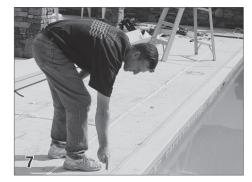
Pull the rope down the back side of the track toward the cover housing.
