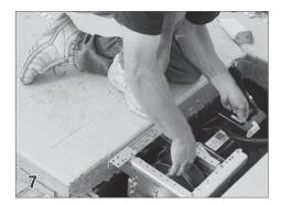
**Positioning the Mechanism** Lower the assembled mechanism and tube into the housing and place it roughly in the position that it will anchored.
