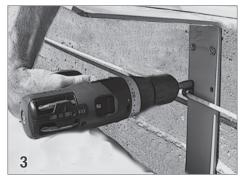
Secure the brackets to the back wall of the housing using  $#12 \times 1-1/2$ " hex head (34) screws. Mount a rope loop (30) on one screw of each of the brackets. This will keep the rope running straight along the back of the housing.
