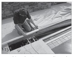
Attaching the Cover Leading Edge Lay the front of the cover in front of the housing. Slide the leading edge through the loop on the front of the cover.
