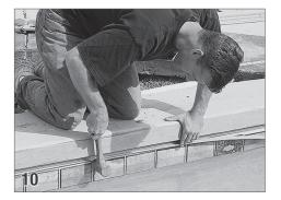
Insert and tap the spacer into place underneath the track along the entire length of the track. Do this along both sides of the pool. The spacer needs to end at the inside edge of the housing
