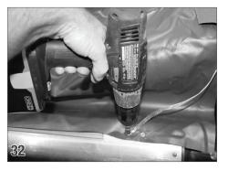
Lay the bond wire on top of the cover fabric. Secure it to the roll-up tube using a tek screw (32). Distribute the slack of the cover evenly between each screw across the length of the tube. Secure the cover to the roll-up tube using tek screws (32) every 2-3 feet. When attaching the cover to the tube, **do not use folds or pleats**.
