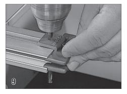
Holding the guide feed firmly, use a 6 inch 3/16'' bit to drill through the hole in the track feed and through the track. Remove the guide feed. Do this for the track on both sides of the pool.
