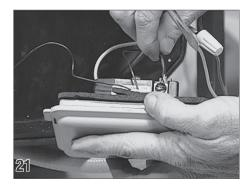
Insert the hot wire from the power supply into terminal L1 on the back of the switch and tighten the screw. Do not loosen the screws too much or the internal switch connections will be permanently lost.
