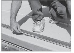
Hold the rope outside the track to pull the rope down the length of the track toward the end of the pool.
