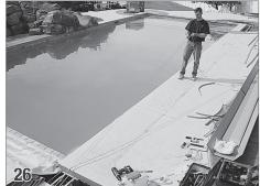
Attaching the Ropes to the Reels Pull the cover back until the sliders are against the stops. Pull the ropes tight as they come off the pulleys on the mechanism to eliminate the slack in the rope.
