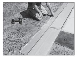
Measure across the hinge to evenly space the screws. Continue drilling and anchoring the hinge in this manner until the entire lid is attached to the deck. The safety pool cover installation is now complete. Now instruct the home owner using the home owner's guide and the checklist on the next page.
