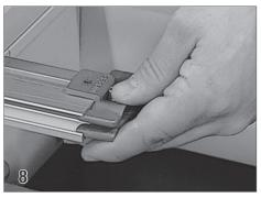
Using a 5/32'' allen wrench, loosen the screw on the top of the guide feed (16). Insert the guide feed on the end of the track that will extend into the housing.
