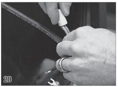
Connect the ground wires from the power supply and the motor together using a wire nut. Run a pig tail from this wire nut to the grounding lug on the switch.
