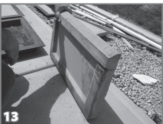
13 The trays were designed so the middle section of the lid will be thinner to reduce the weight of the lid section.
